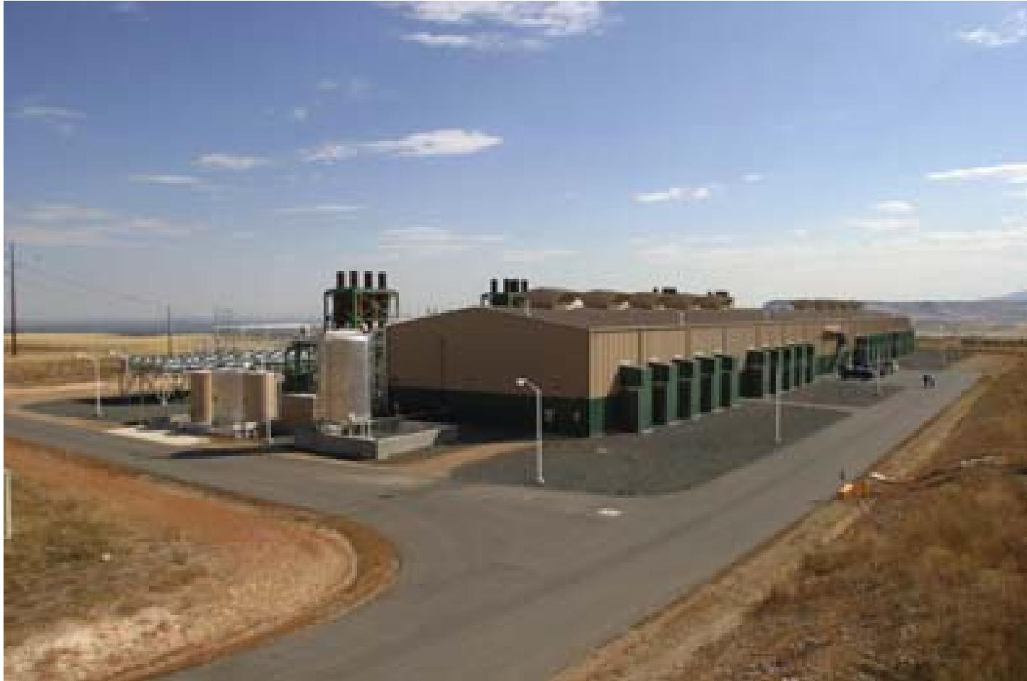
Excel Energy Plains End Generating Station (Colorado)
